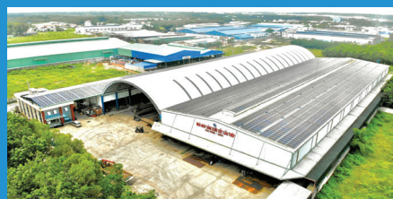
Steel Structure Factory 2 Quarter 4, Vinh Tan Ward, Ho Chi Minh City
